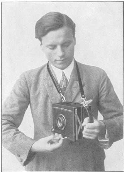
Fig. 2 The Miroflex as a Reflex Camera. Opening the camera
